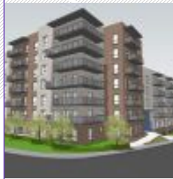
ST ANDREWS PARK, UXBRIDGE
