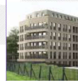
GRANGE ROAD, NEWHAM
