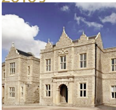
Refurbishment, The Old Hospital, Maidstone
