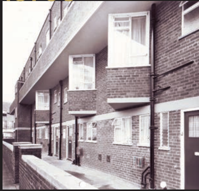
Refurbishment Works, Chelsea Manor Buildings, Chelsea
