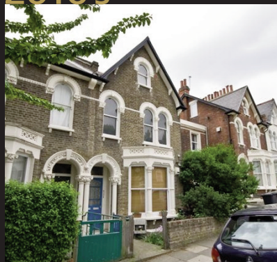
Refurbishment Works, Brockley PFI
